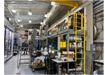
ISU Bioprocessing Plant
